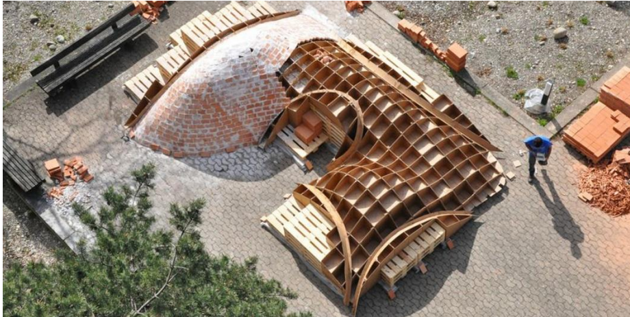
Fig. 1. Free-form Catalan Thin-tile vault, Zurich, Switzerland. BLOCK research group. http://block.arch.ethz.ch/brg/project/free-form-catalan-thin-tile-vault
